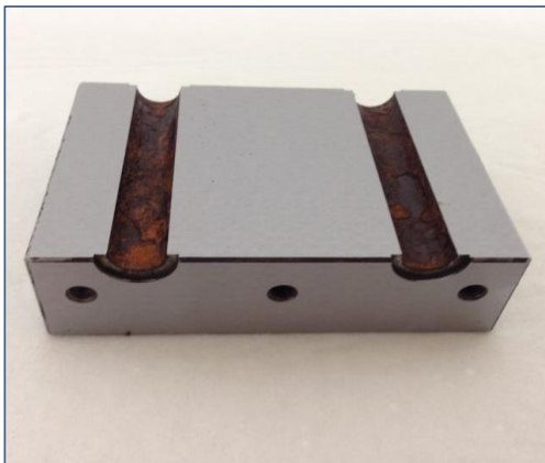
Longitudinal section of cooling pipe before cleaning
